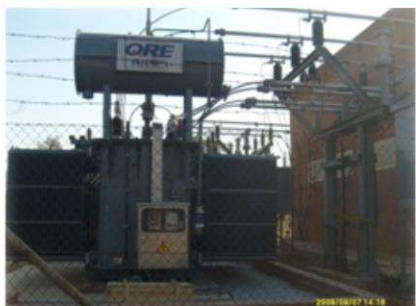
3X 20MVA,33/11kV With OLTC Mokopane Project,South African
