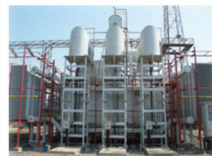
4X40MVA, 90/11kV Power Transformer , Senegal
