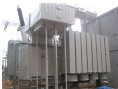
18/23MVA , 230/34.5kVPower Transformer, Keneya
